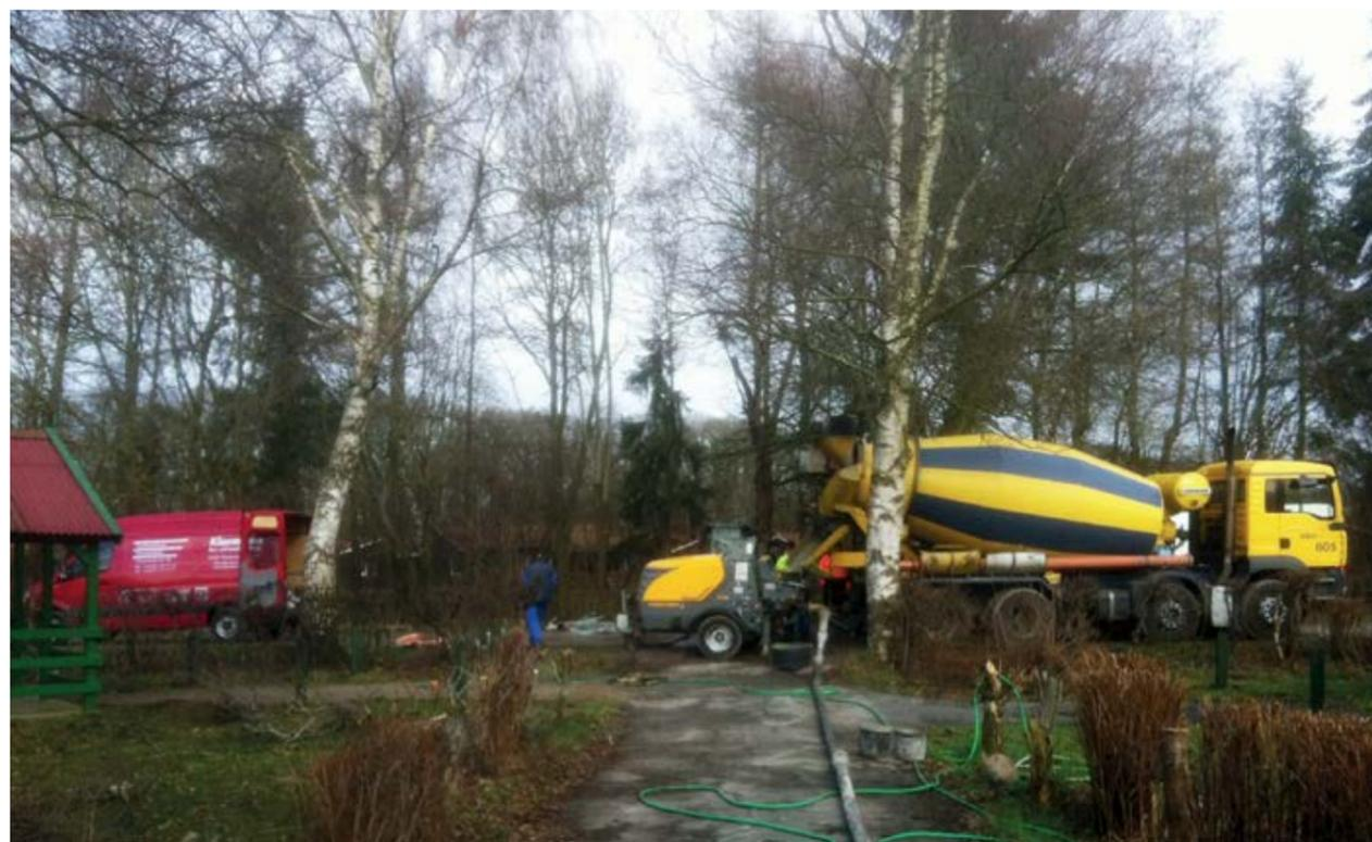
The Putzmeister P 718 pumps concrete through hose lines up to 150 m directly to the site of concrete placement.
